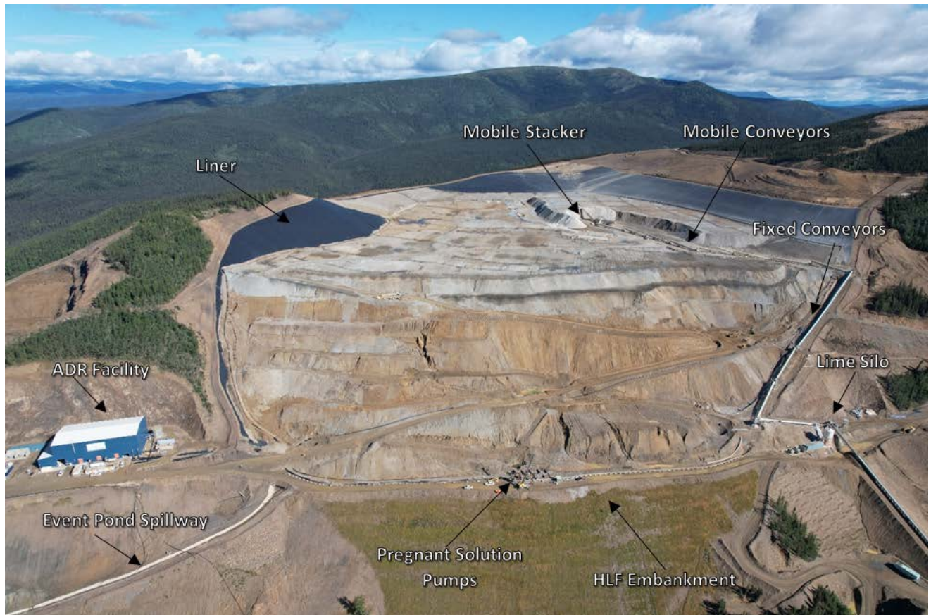
Figure 1: Heap leach facility layout at Victoria Gold Corp.'s Eagle gold mine
