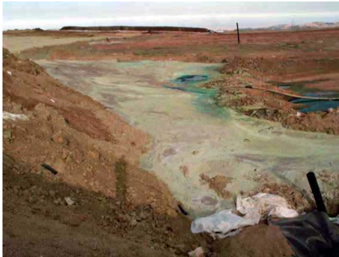
Figure 3: Liquefaction of the Cuajone Copper Heap, Peru
