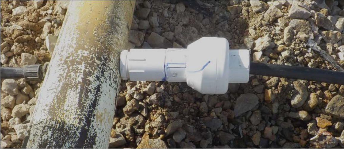
Figure 3: Photograph of the Check excess flow valve
