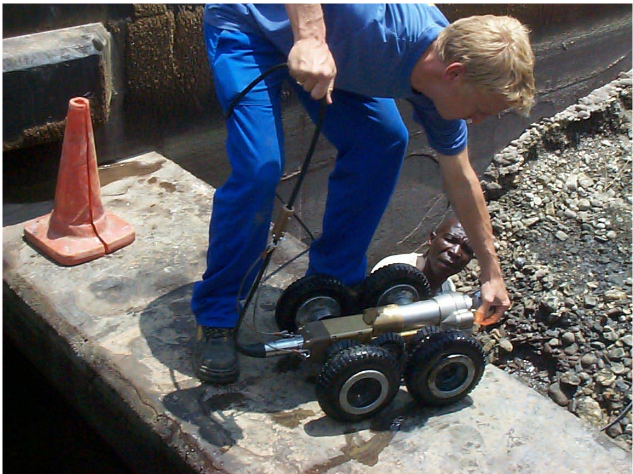
Figure 2: Photograph of camera being used for pipe inspection
