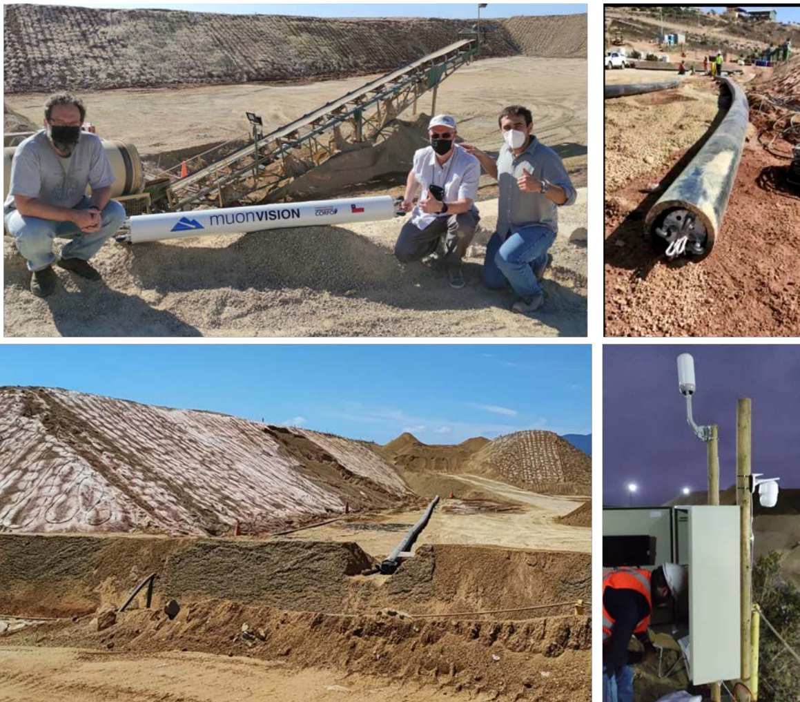
Figure 2: Clockwise from top left: i) the Muon Vision team on site, with the prototype sensor, prior to installation; ii) the Muon Vision sensor inside the HDPE pipe during tests; iii) the remote cabinet for managing power and data connection on site; and iv) overview of the installation pipe, next to an already leached section of the heap, and prior to construction of the heap module measured
