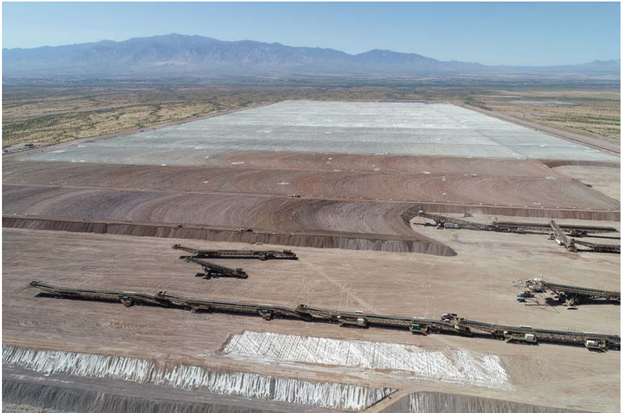
Figure 3: Active stacking of the Lone Star leach pad
