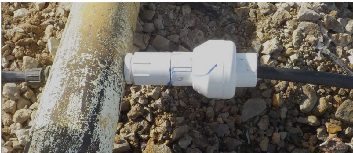
Figure 3: Photograph of the Check excess flow valve
