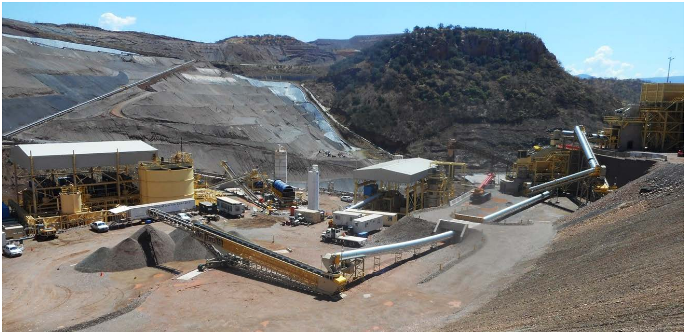
Figure 5: Pan American silver pulp agglomeration mill expansion (designed and built by KCA)
