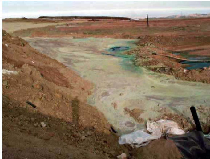
Figure 3: Liquefaction of the Cuajone Copper Heap, Peru
