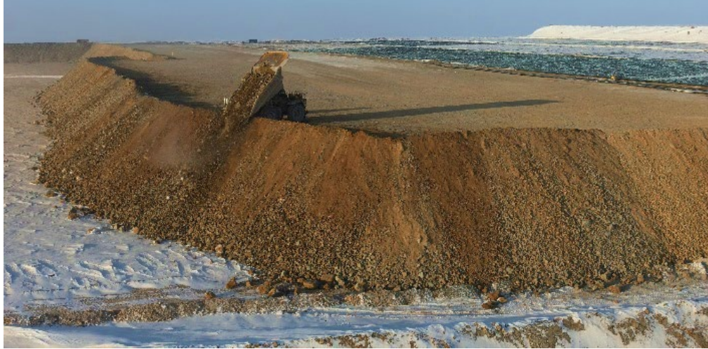
Figure 4: Haul truck end-tipping typical oxide ore (rock fill) on 13 m high lift. Rock fill angle of repose ranging from 37 to 39°
