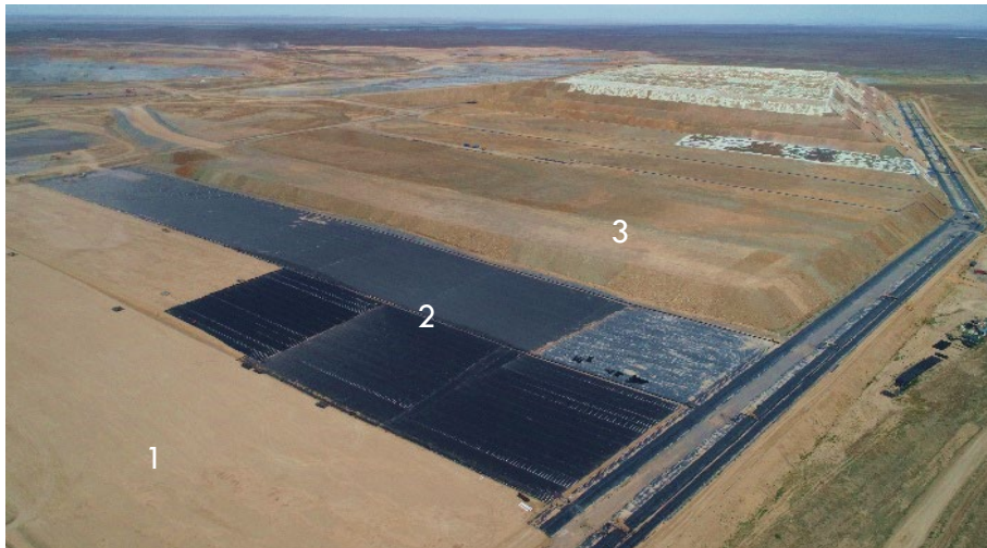
Figure 3: HLP construction sequence. 1: Engineered fill base and clay underliner with \geq 1\% gradient. 2: LLDPE installed on clay under-linear. 3: Coarse overliner and initial oxide ore lift
