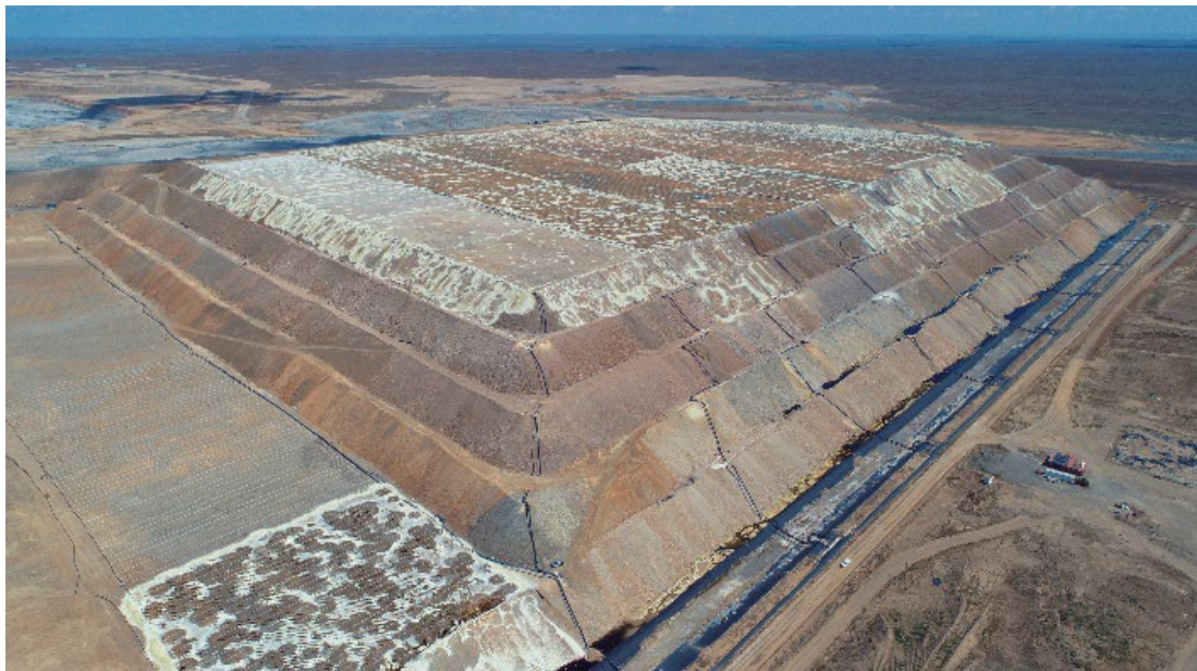
Figure 2: Completed HLP Stage 1: 65 m high (5 lifts)
