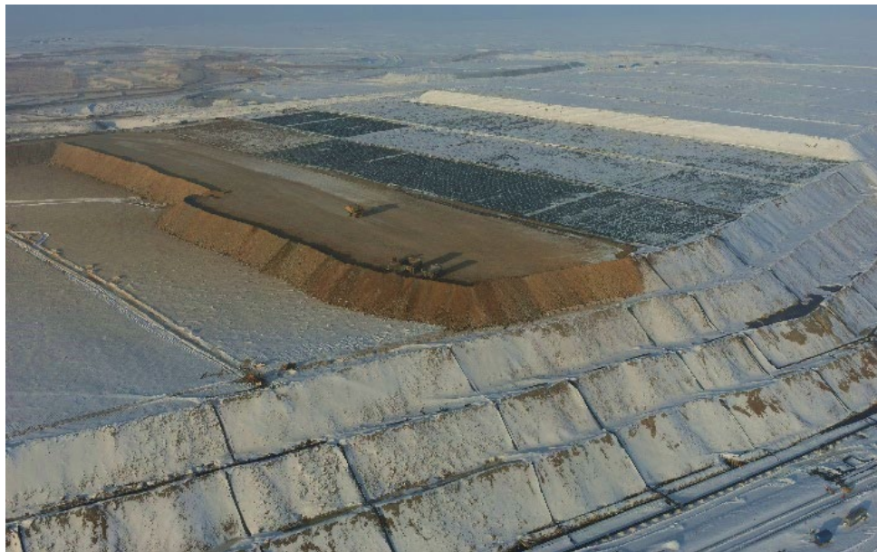
Figure 1: Construction of the Aktogay Copper Mine HLP Stage 1 during winter, Kazakhstan
