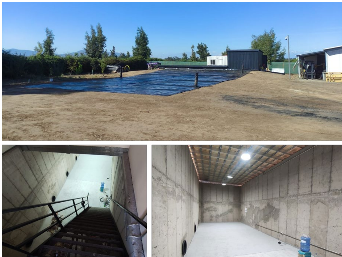
Figure 5: Overview of Muon Vision's demo facility, as built
